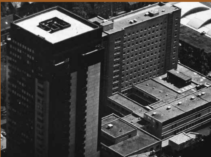
Fig 20 St Gallen hospital in 1960.
