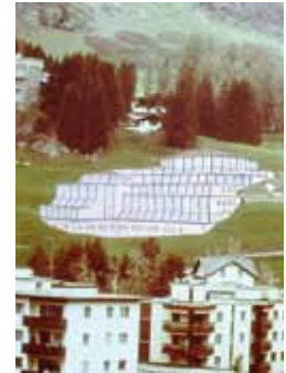
3. An interesting but dangerous location in an avalanche area near the POMD.
